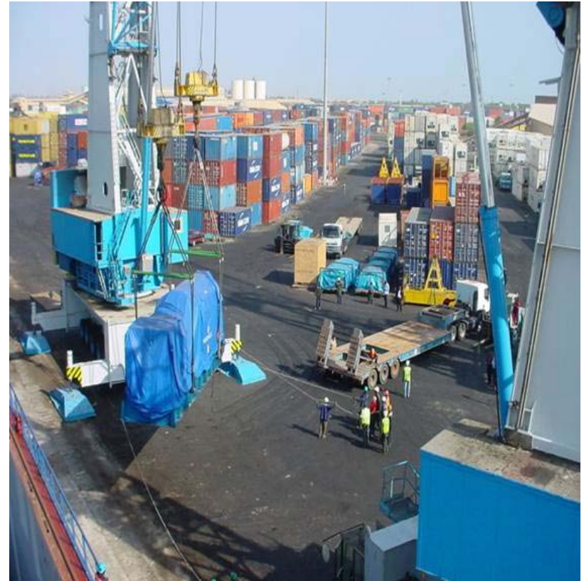
Bank-financed Container Terminal. Dakar, Senegal.
